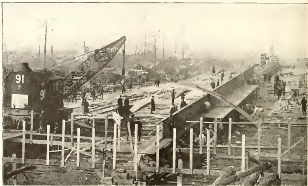
LAYING THE FIRST KEEL, THAT OF THE QUISTCONCK, AT HOG ISLAND, PA., UNDER THE SUPERVISION OF JAMES D. MACBRIDE, '99
